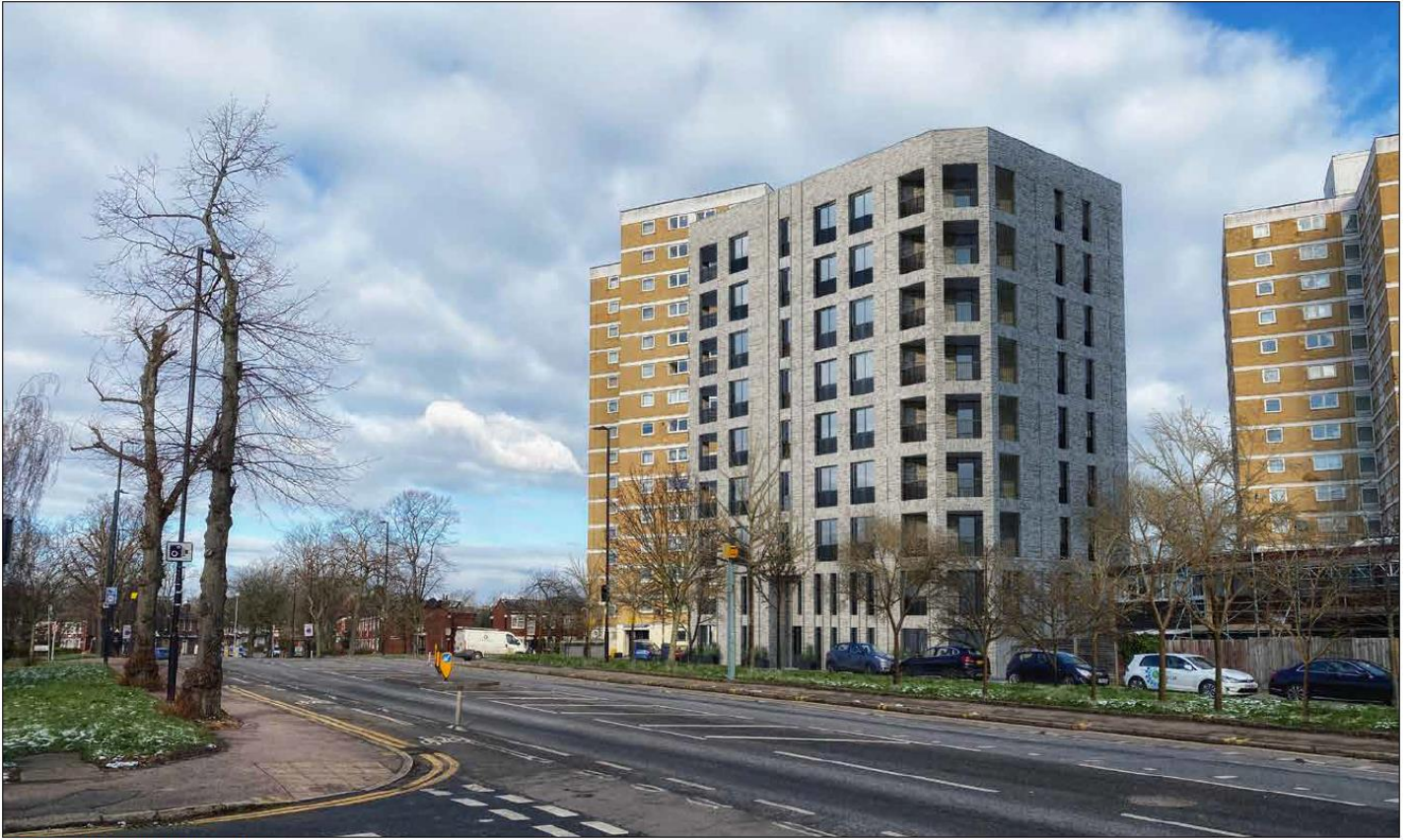
57.2 View looking north on Bounds Green Road
